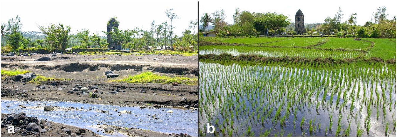
Figure 17: a) Damage above the northern wall surrounding the Cagsawa site shown in Figure 16 ( February 2007). b) The same view following rehabilitated and cropping to rice, January 2009.
