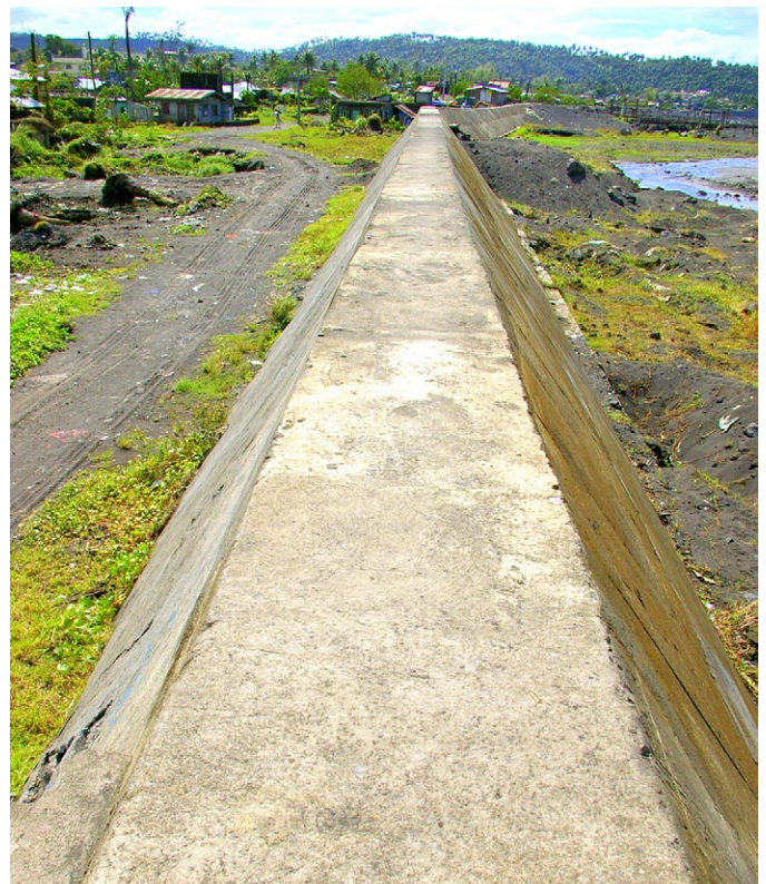
Figure 2: A concrete dike constructed at Daraga in 2007-8 following major loss of life in the 30 November 2006 lahar event.
