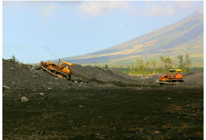
Figure 13: Construction of ash dike in the Lidong area, National Highway (February 2007).
