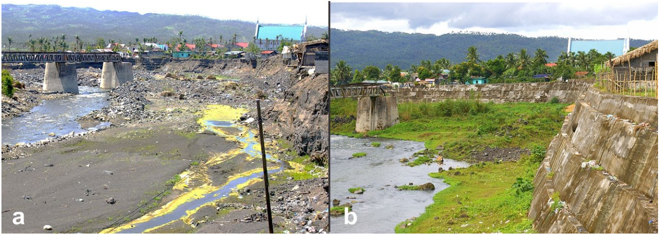
Figure 23: a) Destruction caused along the river passing Guinobatan by lahars on 30 November 2006 (photo February 2007) and b) post concrete sabo construction (January 2009) at the same site.
