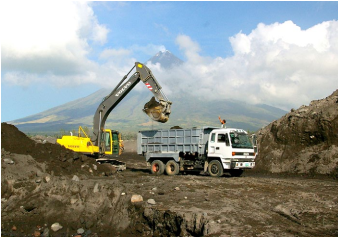
Figure 12: Immediate excavation of an ash-infilled river channel to protect from any new lahar activity, Lidong, February 2007.
