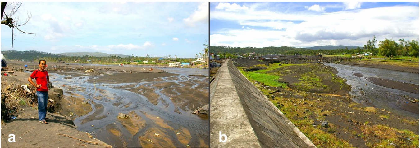
Figure 24: a) Destruction caused along the river passing through Daraga by lahars on 30 November 2006 (photo February 2007) and b) post concrete dike construction (January 2009) at the same site.
