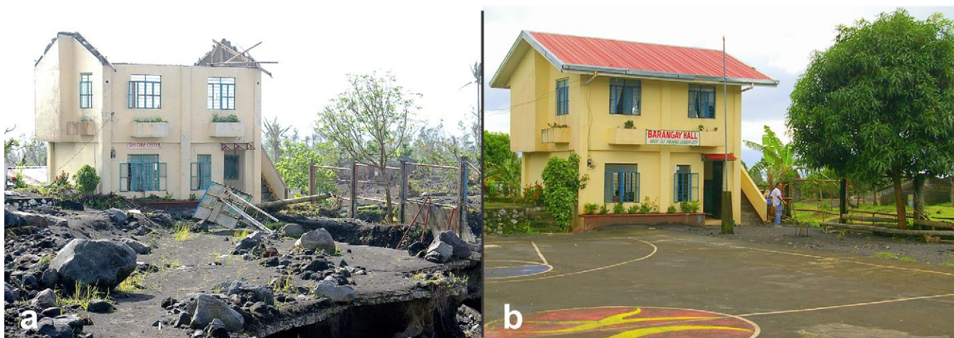
Figure 20: a) This building in Padang doubles as both a Barangay office and a day care centre (photo taken in February 2007), and b) the same building in January 2009.
