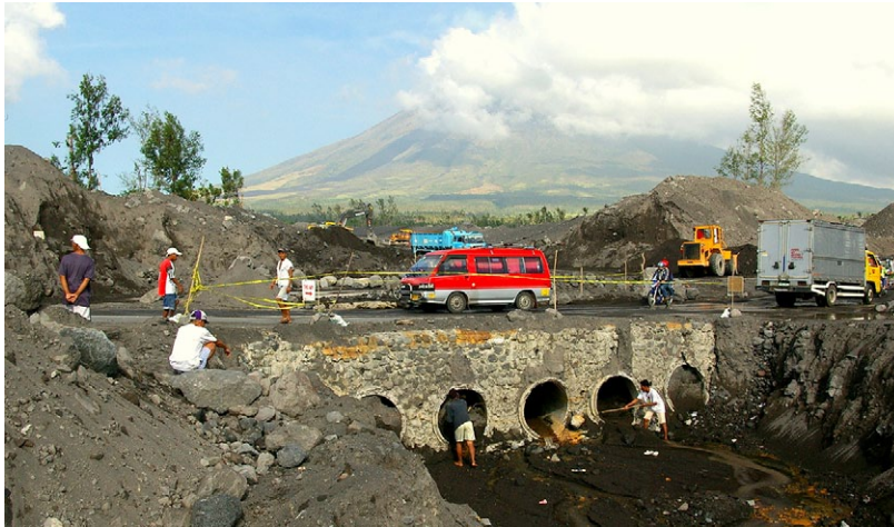
Figure 14: Cleaning ash from an in-filled bridge at Lidong on the National Highway, north of Legaspi (February 2007).
