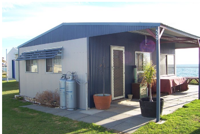
Figure 10: Naval Base post-cyclone rebuild.
