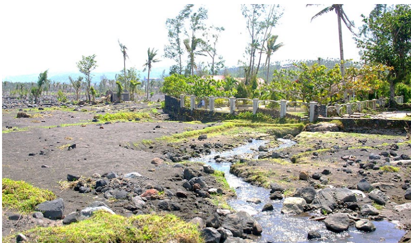
Figure 16: A lahar came up against but did not overtop the retaining wall of the Cagsawa National Museum site and was deflected to the left. A stream has re-established itself and continues ash sediment transport. February 2007.
