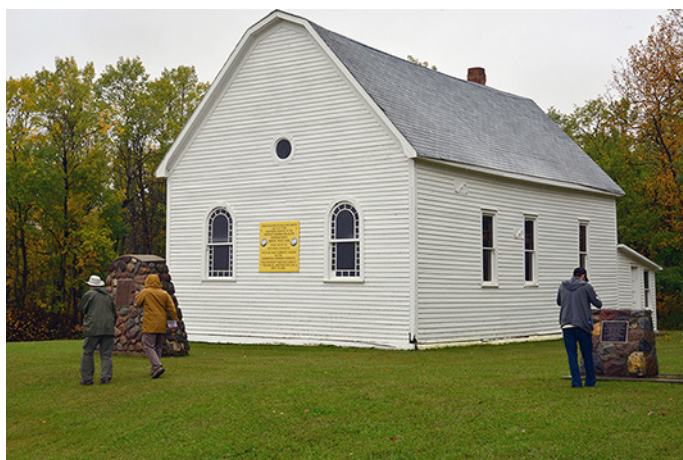
Figure 2 Beth Israel Synagogue Photo credit: Weldon Hiebert
